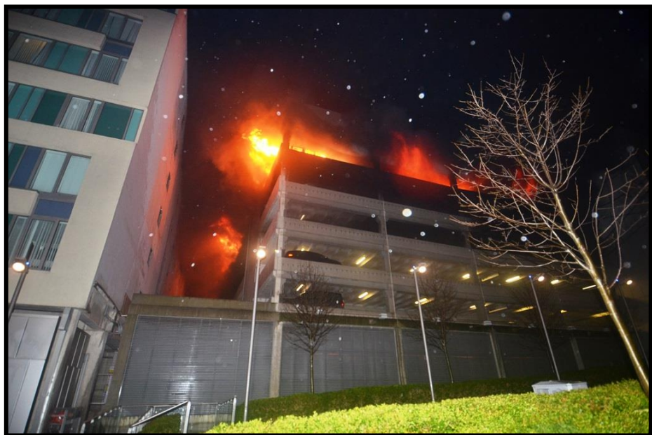
View of fire from opposite main entrance to car park
