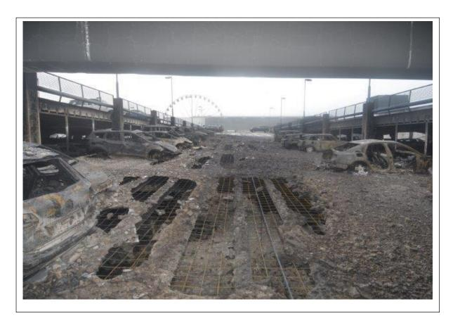
The explosive spalling of the concrete, particularly of the precast ribbed floor slab, may have provided an additional route for fire development between levels. However, the fire severity for this event to occur would be well in excess of the fire design resistance period. The integrity of the concrete and its resistance to spalling will depend on many factors, such as water content; whether the concrete is reinforced and the aggregate and materials used.
