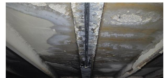
Figure 2.2.6: melted aluminium drainage tray and visible drainage slot
