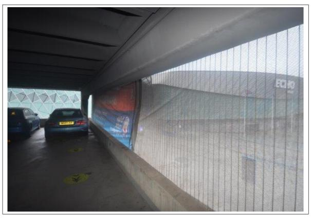
As can be seen from the above photographs (**Figs. 4.1 & 4.2**), the apertures between columns are covered by grilles. These 'Tigris Woven Mesh Panels' cover the apertures from level 3 to level 6 on the northern and western elevations. The free area of these mesh panels is 65 %, according to GKD UK, the PC-Tigris data sheet. This was taken into account by both LCCLABC and MF&RS in their calculations.
