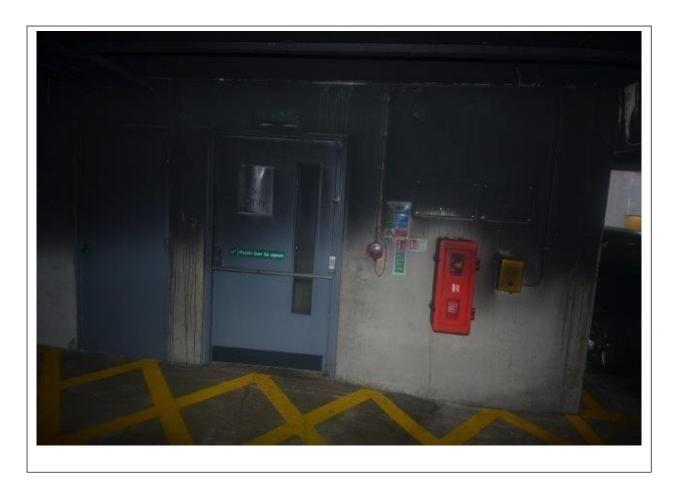
Stairwells 3 and 4 are only available on actuation of the fire alarm. The push bar doors are locked by magnetic devices, linked to the alarm panel. These stairwells are not accessible from outside the car park, for security reasons. Members of the public complained of difficulty in opening the emergency escape door to stairwell 3, level 3.
