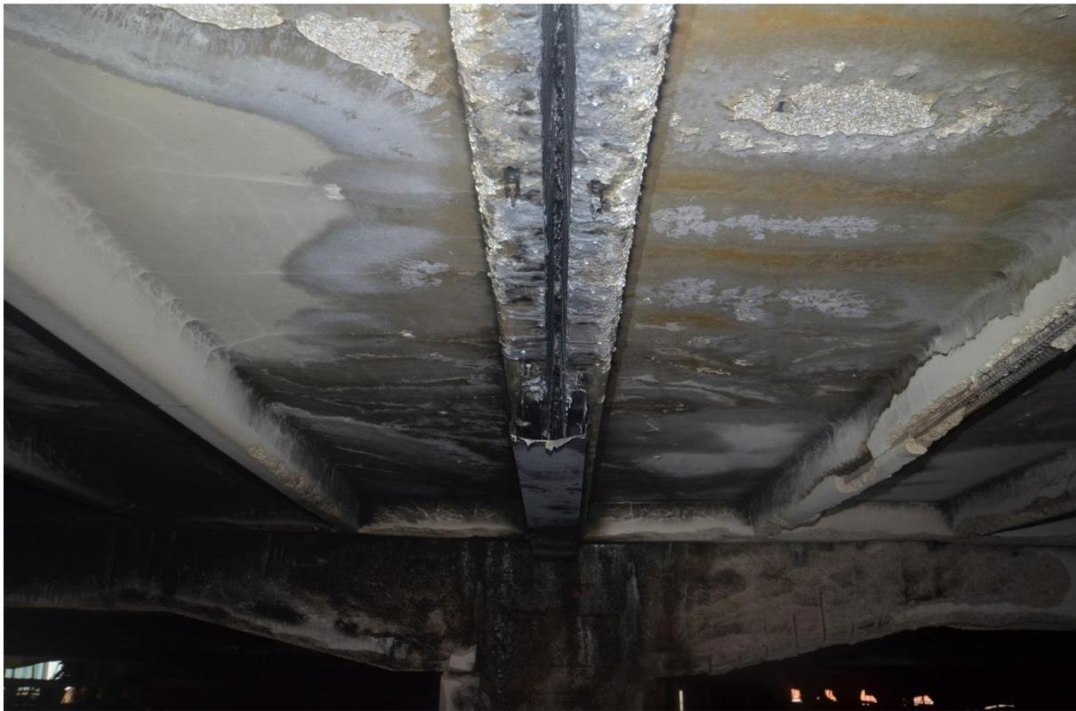
A section of undamaged drainage tray from the car park has undergone testing by BRE. This has confirmed it to be 2mm thick aluminium, which would fail at around 660°C.
