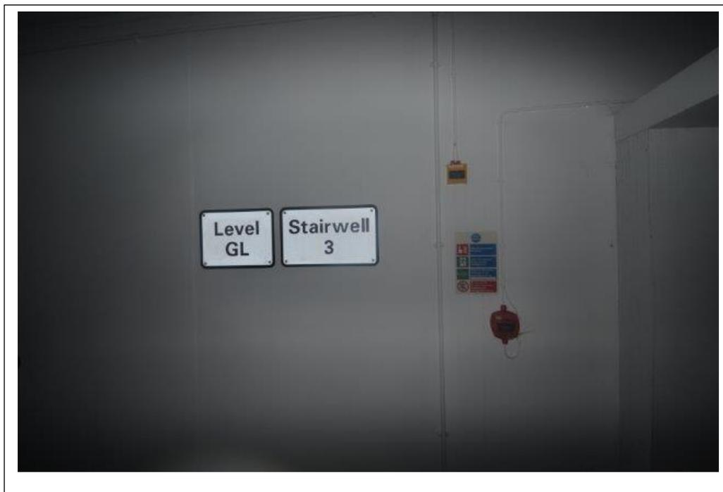
The car park and all escape routes are provided with emergency lighting, conforming to BS5266 and emergency signage conforming to BS5499.
