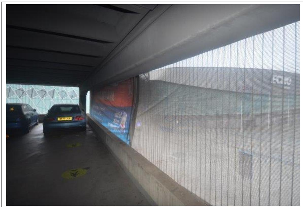
As can be seen from the above photographs (**Figs. 4.1 & 4.2**), the apertures between columns are covered by grilles. These 'Tigris Woven Mesh Panels' cover the apertures from level 3 to level 6 on the northern and western elevations. The free area of these mesh panels is 65 %, according to GKD UK, the PC-Tigris data sheet. This was taken into account by both LCCLABC and MF&RS in their calculations.
