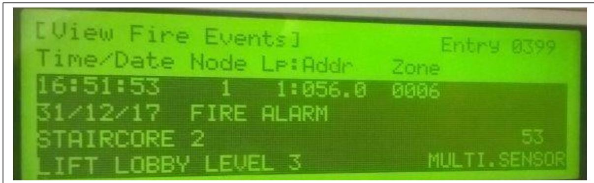
However, the photograph below was taken in the lift lobby area of stairwell 2, level 3 and clearly shows the number 56, once the products of combustion had been removed from the identity label.
