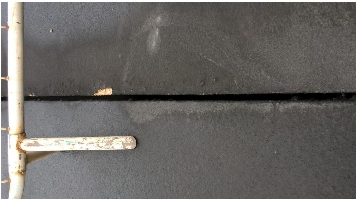
This drainage slot runs between columns with two rows of three cars parked between each column. The drawing below shows the shape of the slot and the guttering below.
